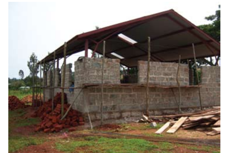
The first home unit - The Penda Home is near completion.
