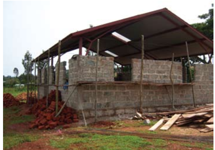
The Penda Home unit nearing completion
